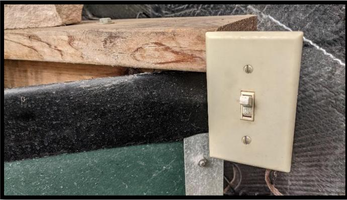
Punch out one of the tabs in the bottom back of the electrical gang box, then feed the wires from the solar panel and the pump through the “tapped” hole in the gang box. You can mount the box on the outside of the pond crossbar or on a nearby strut. There is plenty of cord on the pump for either installation position. Use the attached nails or use two screws to mount the gang box.
