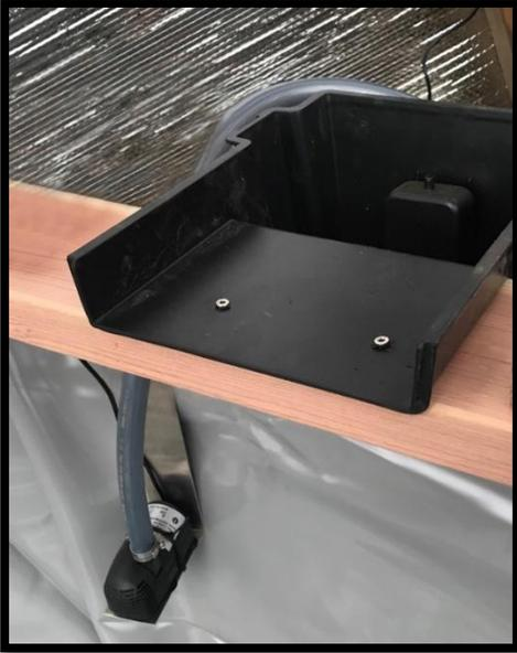
Attach the tubing to the spillway reservoir. Place the spillway towards the center of the crossbar so that the water won't spill out of the pond. Place the 2 composite shims under the spillway to create a slight downward angle. Drill two 3/16" holes through the spillway into the crossbar and place a drop of silicone in the holes. Secure using 1-1/2" stainless steel screws.
