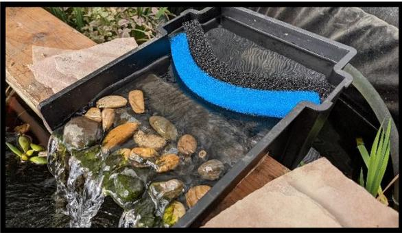
There are 2 filters that come with the spillway kit. Install the course filter in the back and the fine filter in the front of the spillway reservoir. You will need to put a slight bend in the filters to get them to fit. Decorate the spillway to add some beauty to your Above Ground Pond. Your solar waterfall spillway should now be ready to use!
